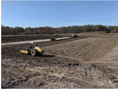
Heavy equipment packs the clay liner to seal the pond.
